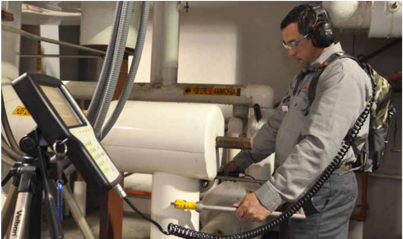
Ingersoll Rand Industrial Refrigeration FHC Facility HealthCheck predictive audit program minimizes potential ammonia leaks into the environment. Submitted by Cheryl Beach, Communications Manager, Industrial Vertical Market, Ingersoll-Rand Industrial Refrigeration, Inc., Bridgeton, Missouri
